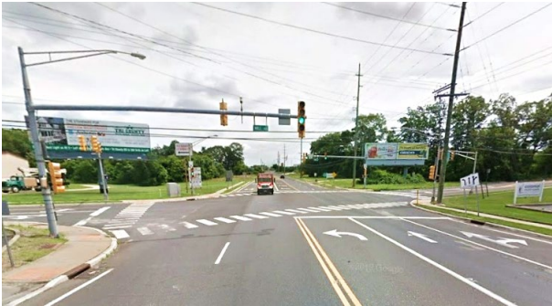
Delilah Road (CR 646) and Mill Road Intersection
